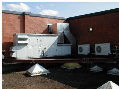
Ducted system with free cooling
