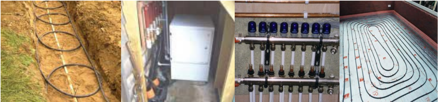
Fig 1: Ground loop being installed to connect to the Heat Pump.
